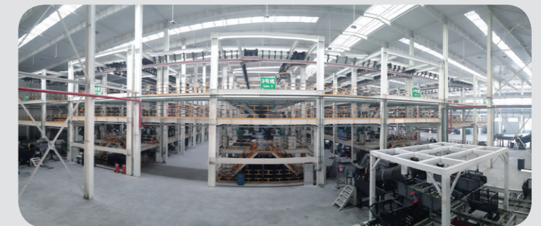
Threading, Air Pressure Test, and Anti-rust Treatment
