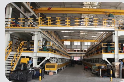
End Grinding Line
